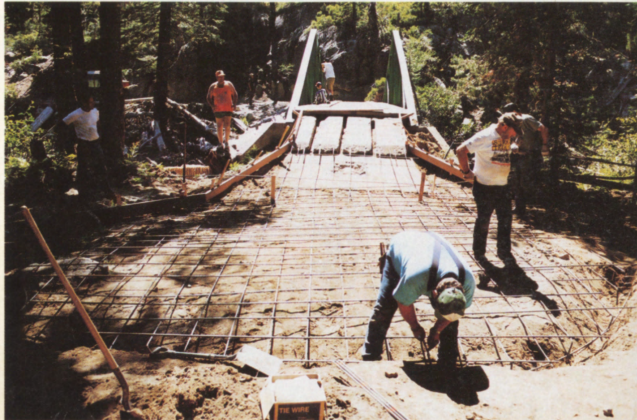
Mike Newcomb tying rebar in preparation for the concrete
