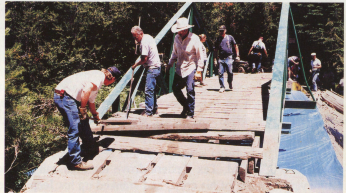
Volunteers stripping the wood planks off the bridge
