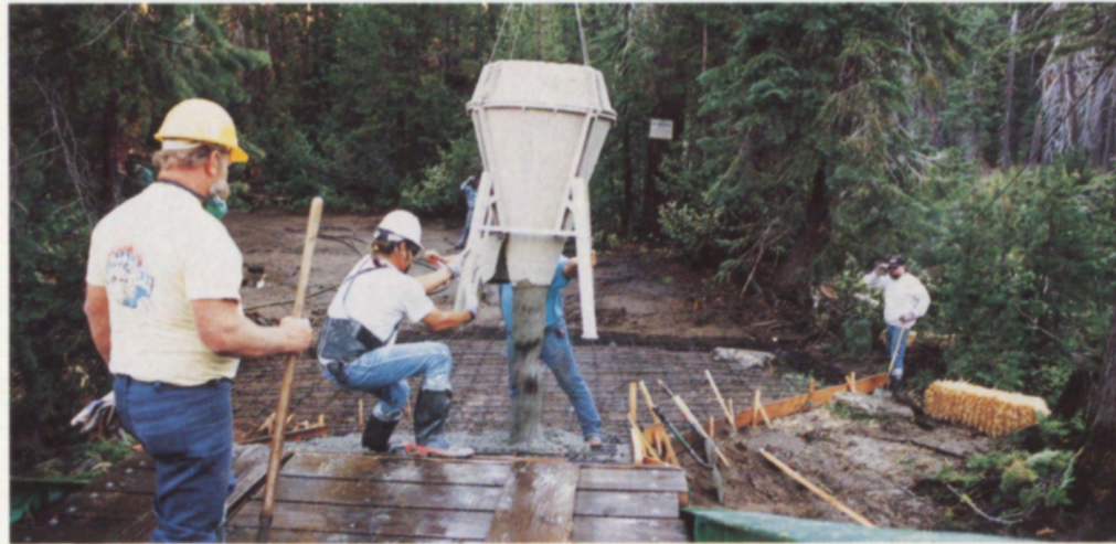
Jack Connelly & Mike Newcomb receiving a load of concrete
