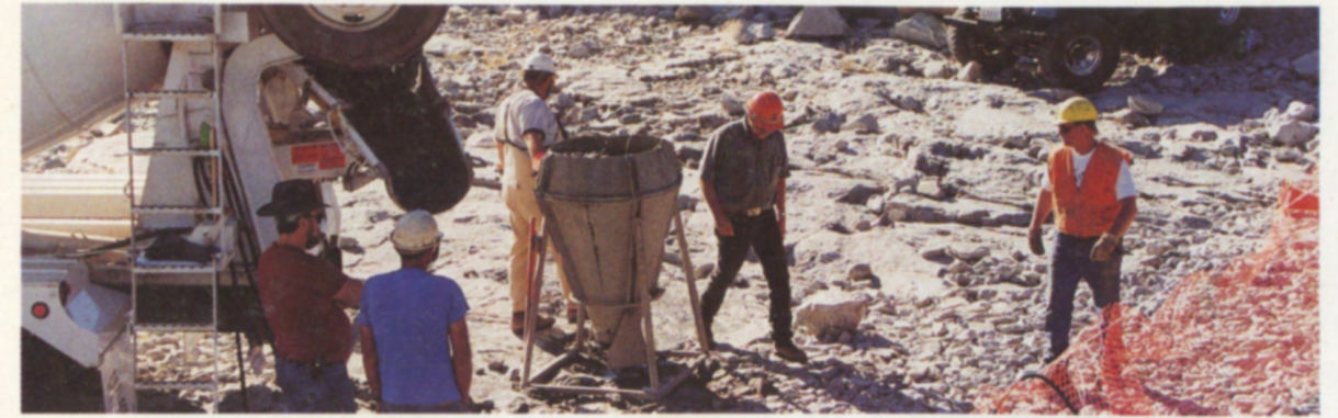
Preparing concrete loads at Loon Lake
