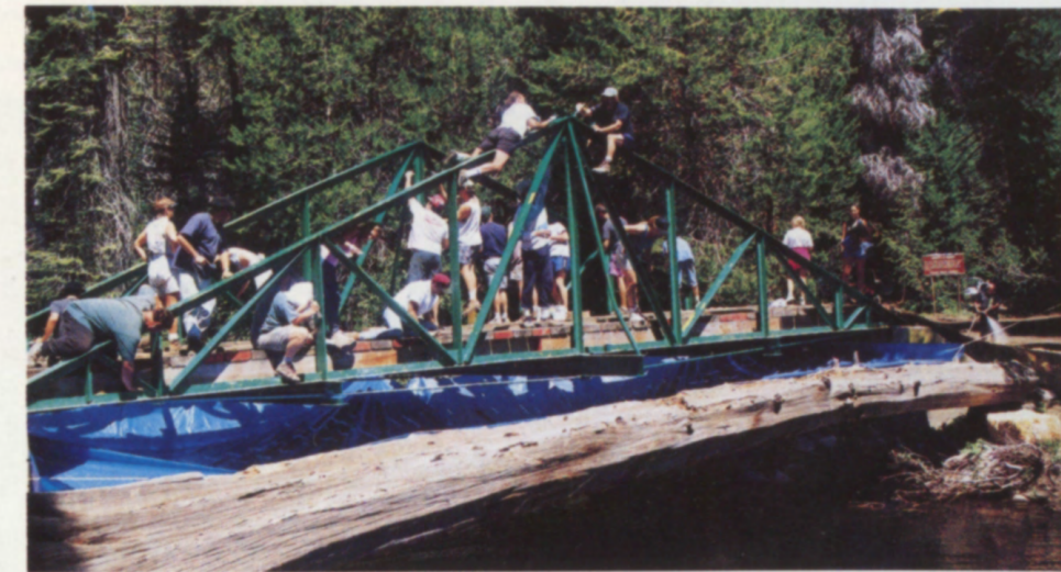
Peninsula Low Rangers painting the bridge
