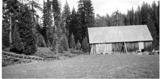
South Fork Sawmill. The penstock at left delivered water from the highline (Sawmill) ditch to the turbine below the main floor of the mill. July 1941.
