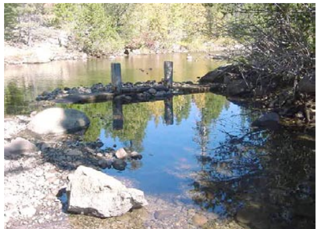
Gerle Creek Ditch, Mile 0.0: Remains of the entrance structure and the two posts mentioned in the Brattland quote. This is the same area shown in the 1936 photo on page 23. October 2001. Photo courtesy of Mike Brattland (via his Gerle Creek History web site).
