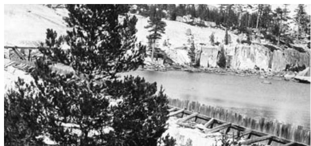
Loon Lake Dam: Probable old quarry area is visible across the lake in this view from the dam left abutment. Photo by California Department of Public Works, Division of Water Resources. August 5, 1930.
