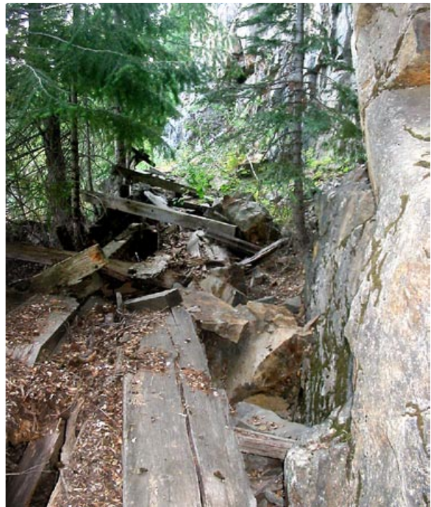
South Fork Ditch, Mile 3.4: Looking upstream back toward the head of the Mile Flume, which is at about Mile 3.35. August 15, 2002.
