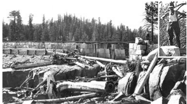
Loon Lake Dam: View of the upstream side of spillway on right (north) abutment, during the 1934 enlargement. Art Rasor (inset) was superintendent on the job. Photo by W.A. Perkins, California Department of Public Works, Division of Water Resources. October 11, 1934.
