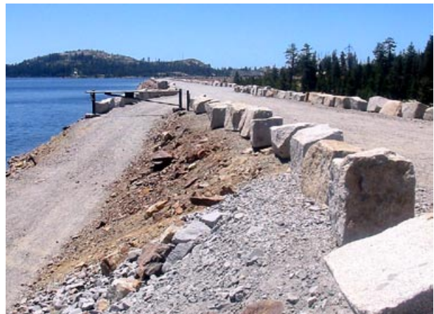
New Loon Lake Dam: Some of the granite blocks from the old dam were set aside for display as sentinels along the roadway on the new dam. June 27, 2002.
