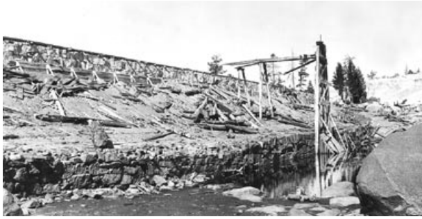
Loon Lake Dam: View from within reservoir area after the 1934 construction. The crumbling tower once provided access to a gatewheel that controlled a headgate on the upstream end of the outlet pipes. Photo by W.A. Perkins, California Department of Public Works, Division of Water Resources. October 11, 1934.
