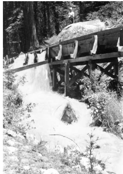
Gerle Creek Ditch, Mile 1.85: The flume to the right led to the South Fork Sawmill. Unless the sawmill was running, all flow was bypassed as shown. (That's me, age 8, up there.) July 1944.
