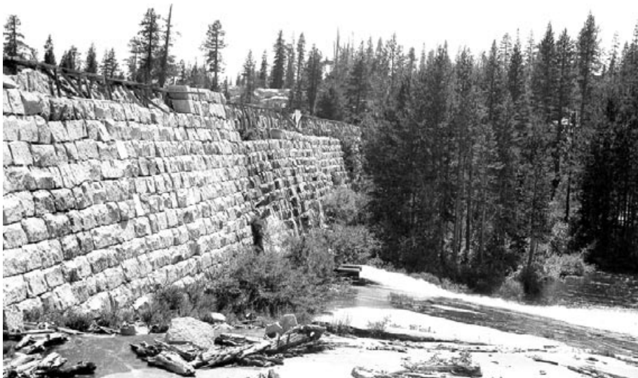
Loon Lake Dam: View from north abutment, showing how the 1934 construction put only one row of blocks on the vertical upstream face. The resulting dam crest was barely 3 feet wide, making for a rather scary walk out to the center of the dam. Photo by David Cleavinger, California Department of Public Works, Division of Water Resources. July 31, 1953.
