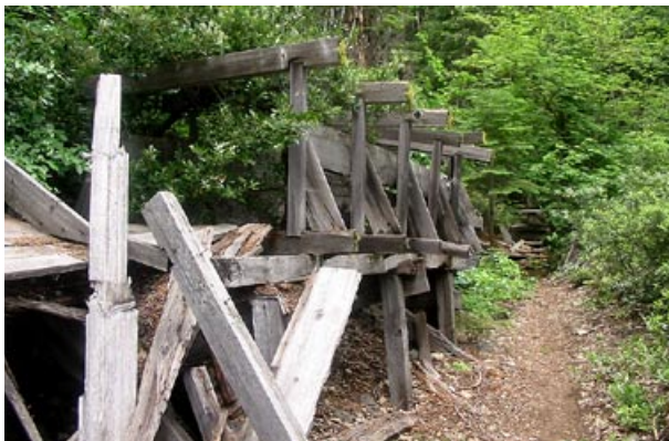
South Fork Ditch, Mile 5.1: Looking downstream at the most intact section of flume remaining. At last we get a feel for what it really looked like! June 26, 2002.
