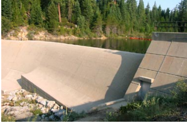
Gerle Creek Ditch, Mile 0.65: The ghost of the old ditch is here somewhere under the left abutment of SMUD's Gerle Creek Dam. August 15, 2002.
