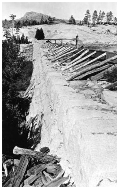
Loon Lake Dam: View from the left (south) abutment, showing the timber parapet wall that was replaced by additional granite blocks in 1934. Photo by California Department of Public Works, Division of Water Resources. August 5, 1930.
