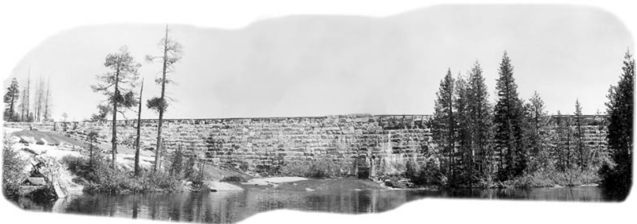
Loon Lake Dam: Panorama of downstream face, showing chronic leakage problem. Lake was 5 feet above the spillway lip at this time. A composite of three photos by Eugene V. Poe, California Department of Public Works, Division of Water Resources. July 3, 1953.
