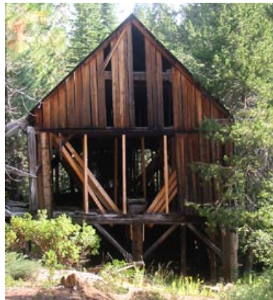
South end of South Fork Sawmill, showing diagonal bracing recently installed by Denton Beam. The turbine was on the lower level. August 15, 2002.
