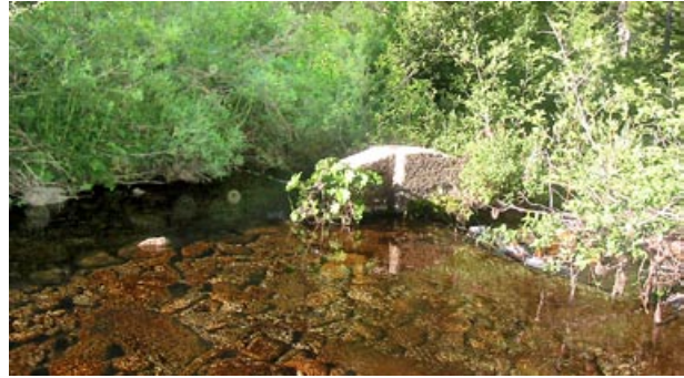
South Fork Ditch, Mile 0.0: One of the four or five piers of the diversion dam on the South Fork Rubicon River. June 27, 2002. Wooden flashboards fit against the indentation on the pier, held in place by water.
