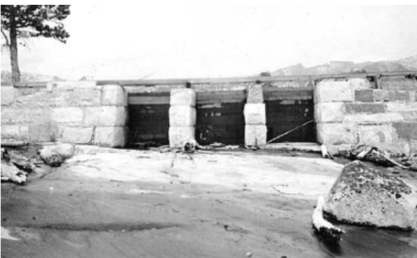
Loon Lake Dam: Spillway on right abutment, with a full complement of flashboards raising the lake almost to the dam crest. Photo by W.A. Perkins, California Department of Public Works, Division of Water Resources. July 12, 1937.
