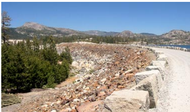
New Loon Lake: Saddle dam at lake's southwest corner, with granite blocks from old dam. June 27, 2002.
