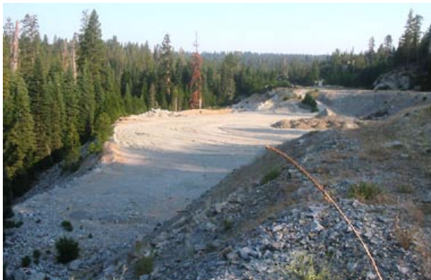
Gerle Creek Ditch, Mile 1.1: Looking northwest along the Gerle Creek Canal toward Gerle Creek Dam. The old ditch is under this filled area. August 15, 2002.
