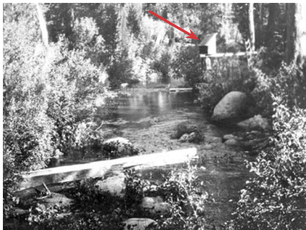
The recorder house for the gaging station, "Little South Fork of Rubicon River at Sawmill near Quintette," operated February 1, 1910 through July 4, 1914 by Stone and Webster Engineering Corp., is still there in this July 1932 photo. The view is upstream on the river, from the bend just upstream from the South Fork Ditch flume, near the old South Fork Campground.
