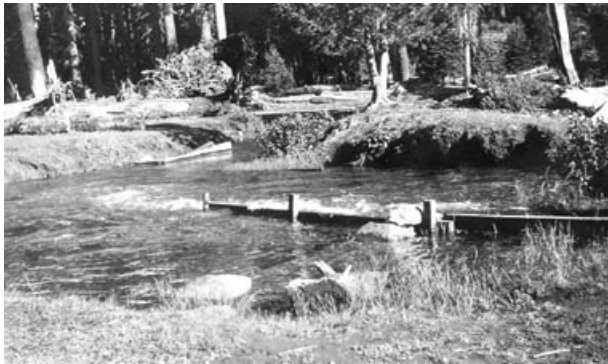
South Fork Ditch, Mile 0.59: Pool at downstream end of the flume at South Fork Campground. June 1932.
