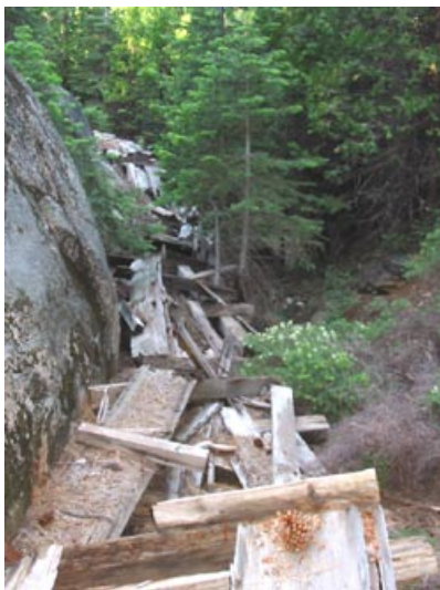
Gerle Creek Ditch, Mile 1.85: This "highline" flume may need a few repairs before it's ready to power the South Fork Sawmill back to life. August 15, 2002.
