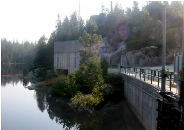
Gerle Creek Ditch, Mile 0.65: Looking from left abutment of Gerle Creek Dam at (left) downstream portal of Loon Lake Powerhouse Tailrace Tunnel and (right) headworks of Gerle Creek Canal. August 15, 2002.
