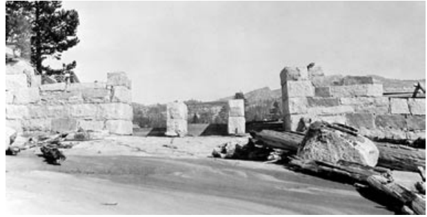
Loon Lake Dam: Downstream side of spillway—showing a few of the wooden flashboards used to increase storage in the spring. Granite blocks were added to the piers in 1934 (below). Photo by H.R. Howells, California Department of Public Works, Division of Water Resources. September 1, 1932.
