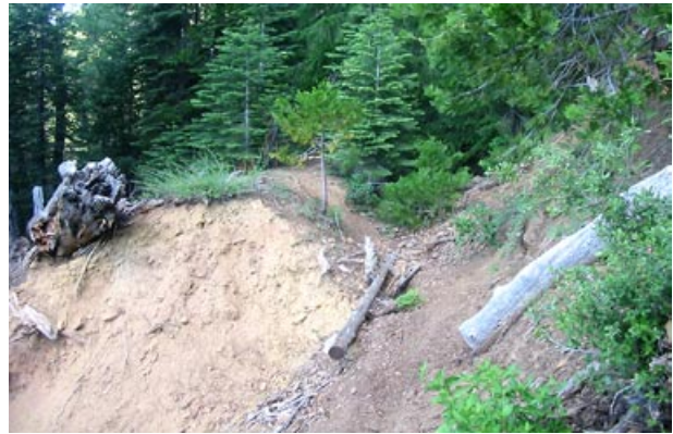
South Fork Ditch, Mile 6.7: The washout that separates the relatively undisturbed ditch from the portion that has been made into a road. June 28, 2002.
