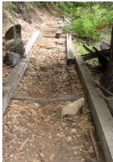
South Fork Ditch, Mile 5.4: A section of flume founded directly on the ground. The flume debris has been pushed over the hillside to open up the trail. June 26, 2002.
