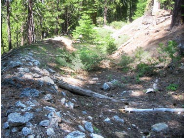
South Fork Ditch, Mile 1.3: Looking upstream about 500 feet east of South Fork Road. June 27, 2002.
