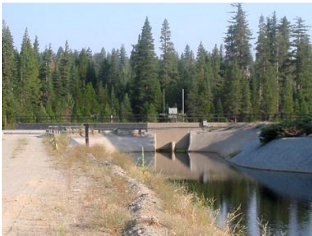
Gerle Creek Ditch, Mile 0.68: Looking back upstream along the Gerle Creek Canal toward the headworks at Gerle Creek Dam. August 15, 2002.
