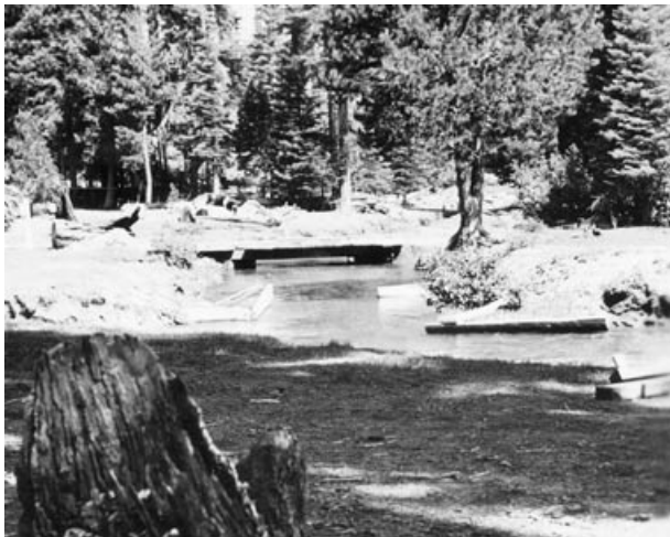
South Fork Ditch, Mile 0.61: Looking downstream at the Wentworth Springs Road bridge, at east edge of South Fork Campground. June 1935.
