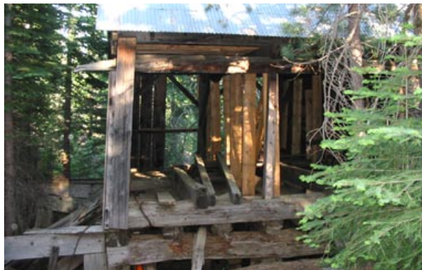
North end of South Fork Sawmill, showing some of the deteriorating supporting members. This is where the logs were rolled in, as shown in the 1956 picture on page 37. June 19, 2002.
