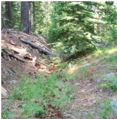
South Fork Ditch, Mile 1.5: Looking downstream at one of the more open areas of this overgrown reach. August 15, 2002.
