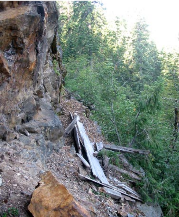
South Fork Ditch, Mile 3.45: Looking downstream. Right around the corner is the end of the trail for the casual hiker. August 15, 2002.
