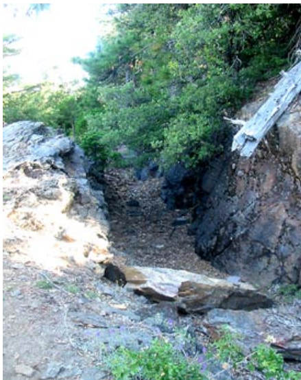
South Fork Ditch, Mile 6.6: Excavated from hard rock, this is about the narrowest section of the entire ditch. June 28, 2002.
