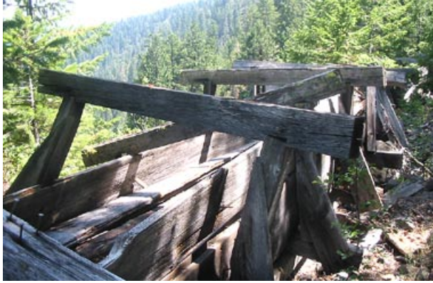
South Fork Ditch, Mile 4.33: Near downstream end of the Mile Flume, just east of the foot of the access trail—the first reasonably intact flume remnant. This is where I made the measurements for the flume section shown as Figure 3. August 15, 2002.
