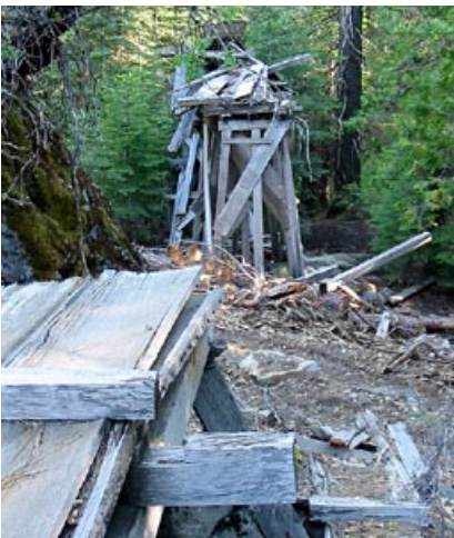
Sawmill Ditch looking downstream (south) at the headworks of the penstock that led to the sawmill. This flume was smaller than the standard design because only part of the ditch flow went to the sawmill. June 19, 2002.
