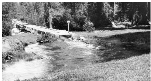
South Fork Ditch, Mile 0.59: The downstream end of the flume over the South Fork. June 1932. The sign probably says "Keep Off," but it wasn't there in later years (not that I'd have paid any attention to it).
