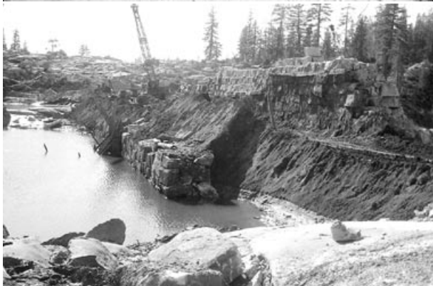
Loon Lake Dam: The end of an era. SMUD's contractor begins demolition of the old dam, in preparation for construction of the new, larger dam in 1963. Photo by Eugene V. Poe, California Department of Water Resources, Division of Safety of Dams. October 30, 1962.
