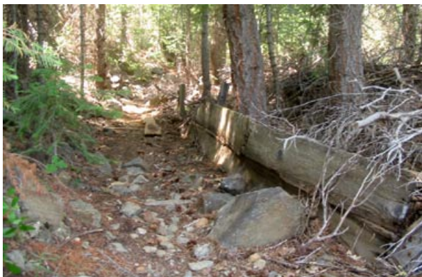
South Fork Ditch, Mile 4.8: Looking downstream. Soil was probably tamped behind the planks to reduce leakage through the rocky bank. August 15, 2002.
