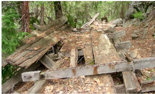
South Fork Ditch, Mile 5.3: Looking upstream, close to the site of Bob's Cabin. June 26, 2002.
