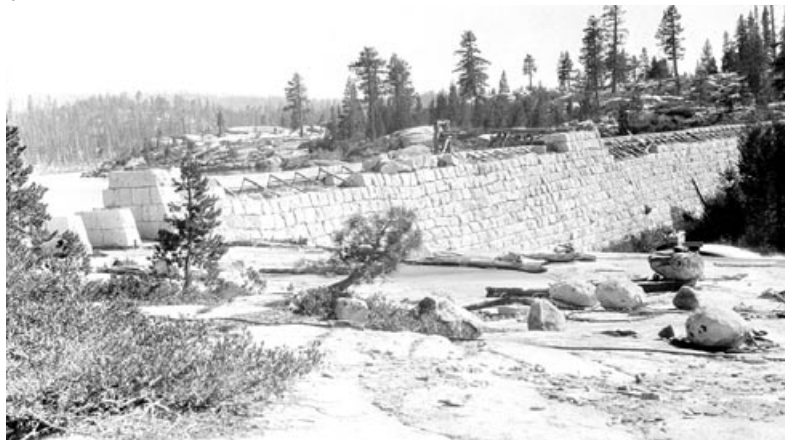
Loon Lake Dam: View from north abutment, showing timber parapet wall installed to compensate for incomplete placement of granite blocks during 1887 construction. Photo by H.R. Howells, California Dept. of Public Works, Div. of Water Resources. September 1, 1932.
