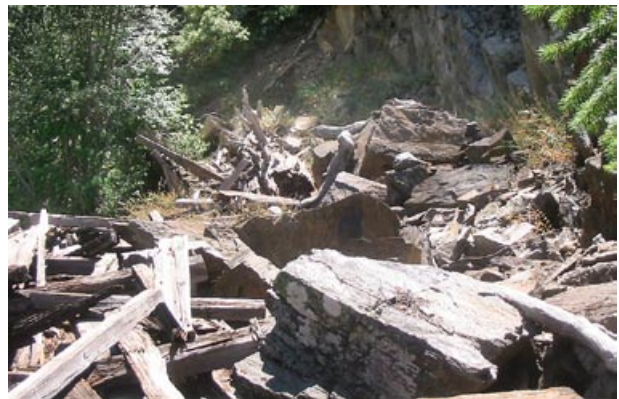
South Fork Ditch, Mile 4.25: The end of the trail when hiking back upstream on the Mile flume. It's easy to see why this section was a maintenance problem during the 87 years the ditch operated. August 15, 2002.
