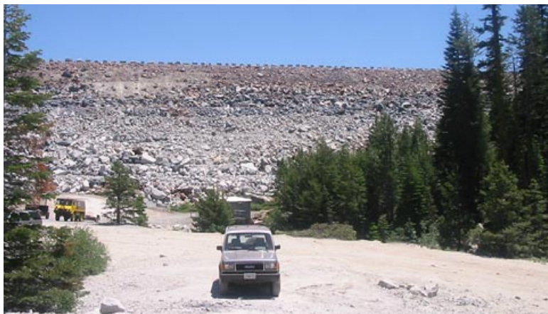
Loon Lake Dam today: just an ugly pile of rocks. The creek outlet is directly above the gray Isuzu. June 27, 2002. The grove of trees on the right is the same one shown on the 1953 photo on page 43.
