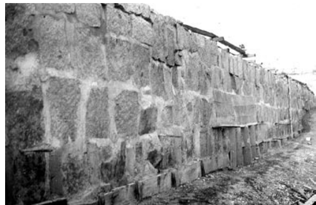
Loon Lake Dam: Upstream face showing repointing of joints to reduce leakage. Photo by Elmer W. Stroppini, California Department of Public Works, Division of Water Resources. November 9, 1953.
