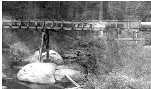
South Fork Ditch, Mile 0.56: Flume over the South Fork Rubicon River, looking south from the Wentworth Springs Road bridge, about 1944. [from the collection of Dale Rasor, Jr.]
