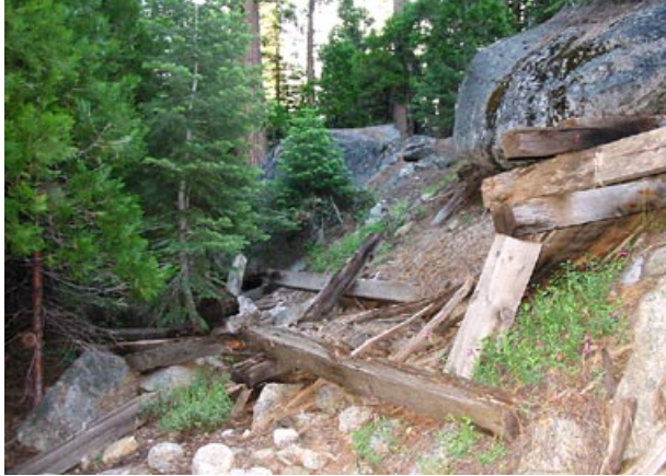
Gerle Creek Ditch, Mile 1.85: Site of the flume spill pictured on pages 24 and 34. August 15, 2002.
