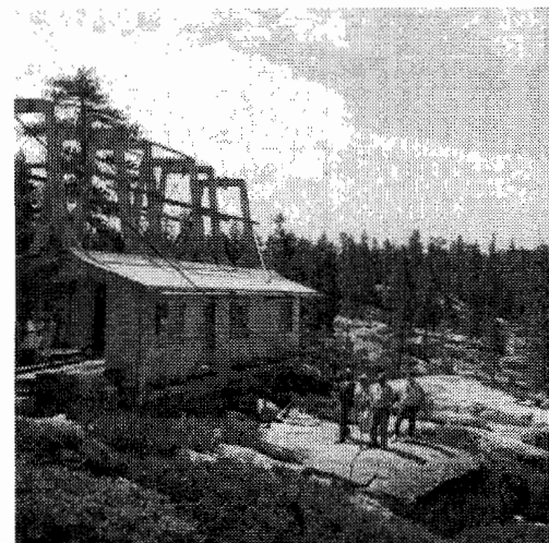
Loon Lake under Construction, 1965.
